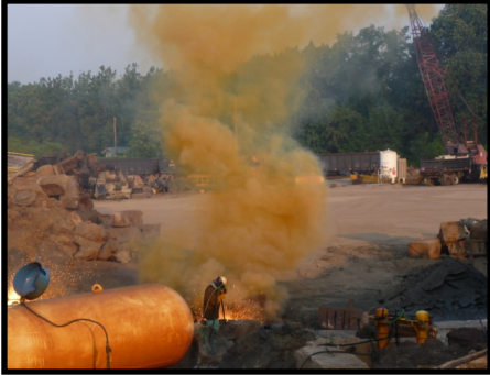
Facility before installing controls
